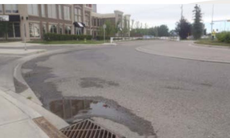
Photo 1 Pavement and stormwater drain
